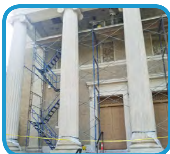
To repair the soffit, a metal work scaffold was erected, including a temporary access stair.
